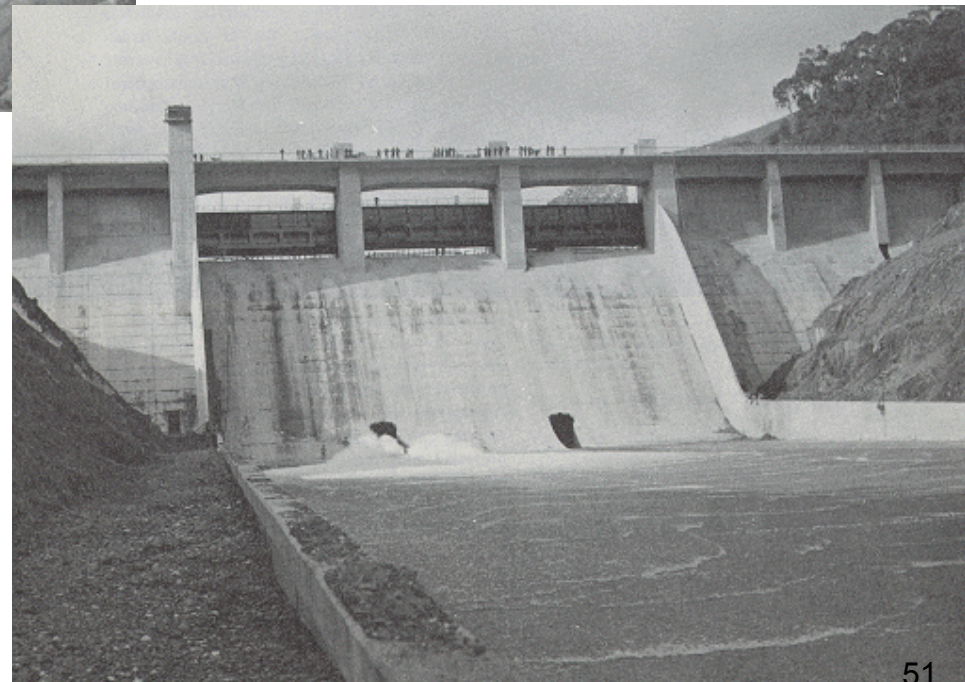
Eildon Dam, Australia
